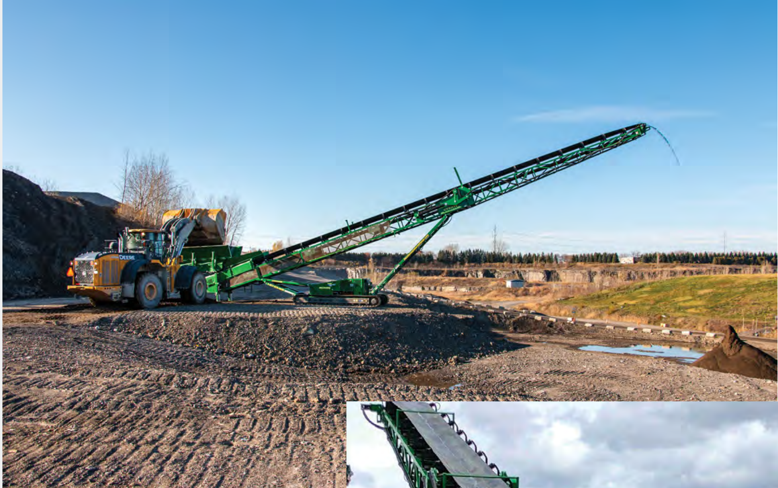
^ ST80TF conveyor Soil reclamation
